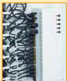
Y-Leads and power pack shelves for improved cable management
